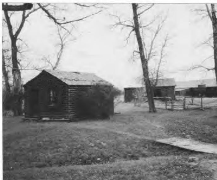
Go across the back yard and over the little bridge...to the office for Montana Knits and Pioneer Mountain Farm.
